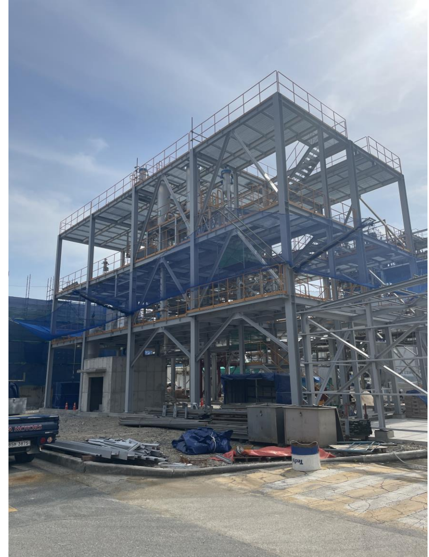
Hysung Chemical EPC for PO Pilot Plant Ulsan, Korea (Ongoing)
